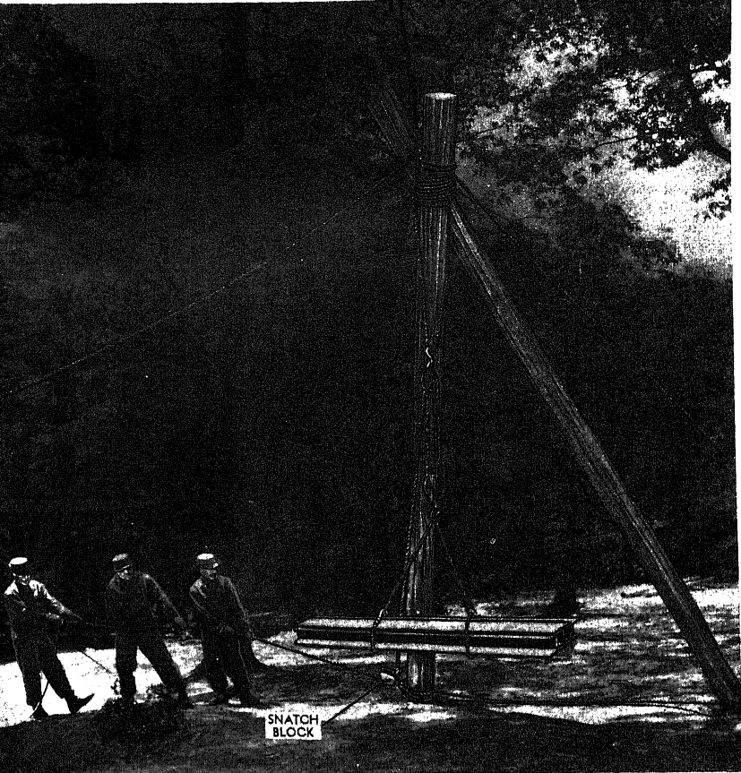
Figure 5-8. Hoisting with shears.
