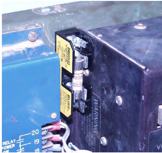
Figure 2. Fuse Holder Orientation
