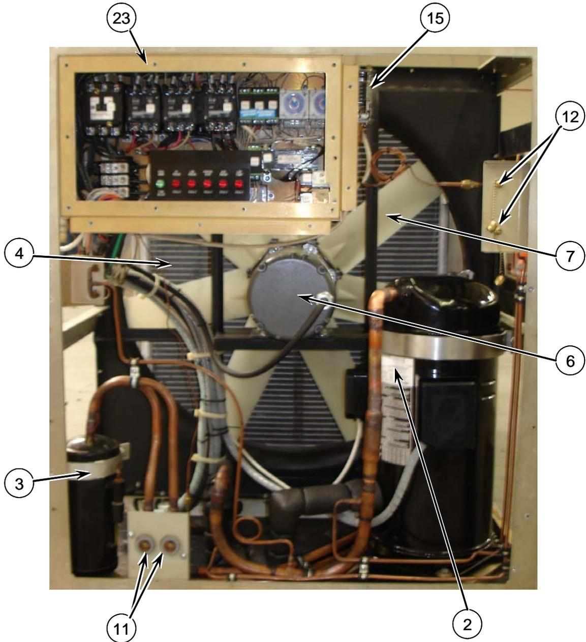
**Figure 8-2 Condenser Side Components, Forward**
